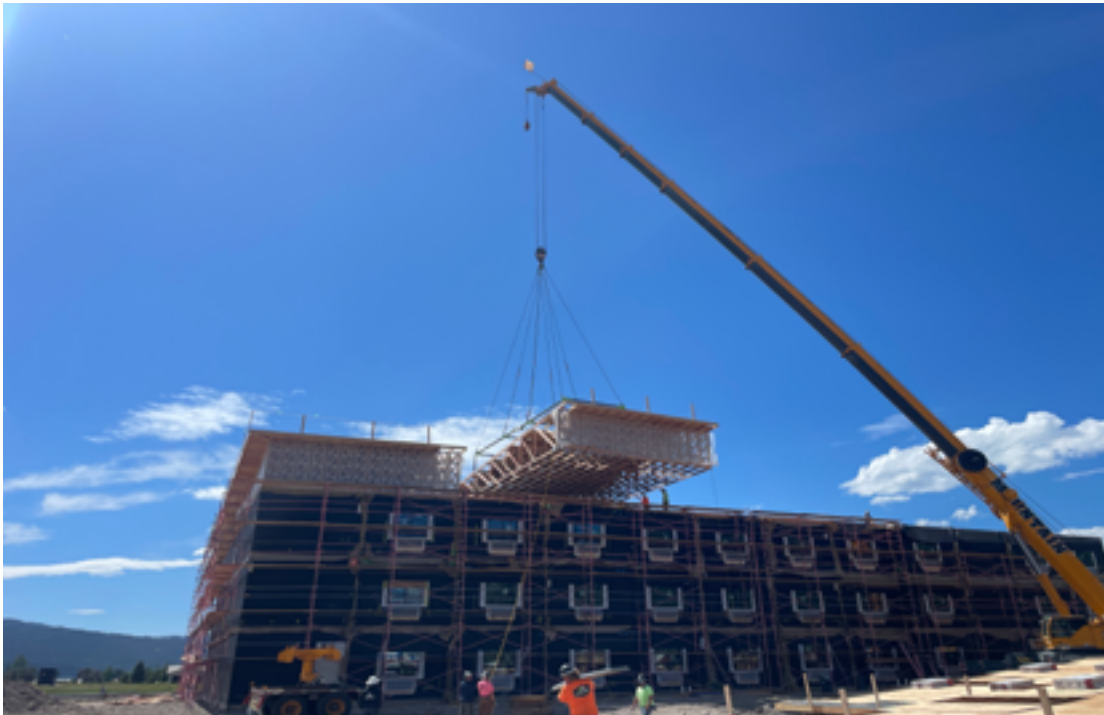
Top: Steve Clough, Autovol Director of Preconstruction Above: The onsite team had these roof pieces ready in advance, so they could be placed by crane very quickly
